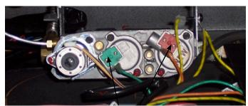
ON/OFF Connector Wires
