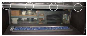
Loosen screw securing the panel clip located in the middle of the side panel - inside the firebox.
