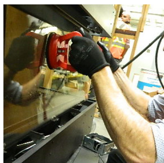
Handle glass with supplied vacuum clamps
