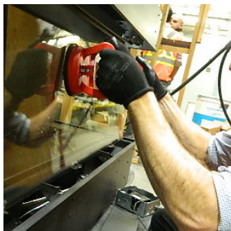
Handle glass with supplied vacuum clamps
