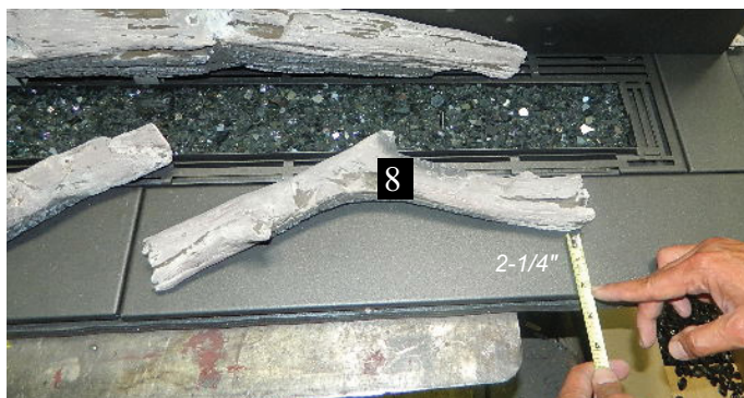
Right end of Log 8--2-1/4" from edge of panel
